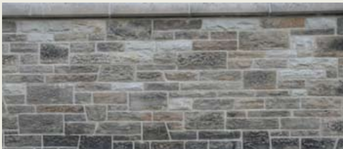
Stone replacements and repointing - Hart House U of T, Toronto.
