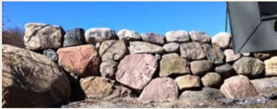
Dry stone retaining wall - Private residence, Port Hope.
