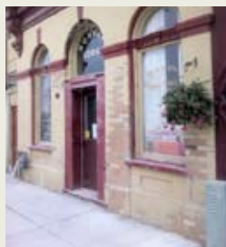
Brick replacements, prepaint- Office facade, Millbrook.
